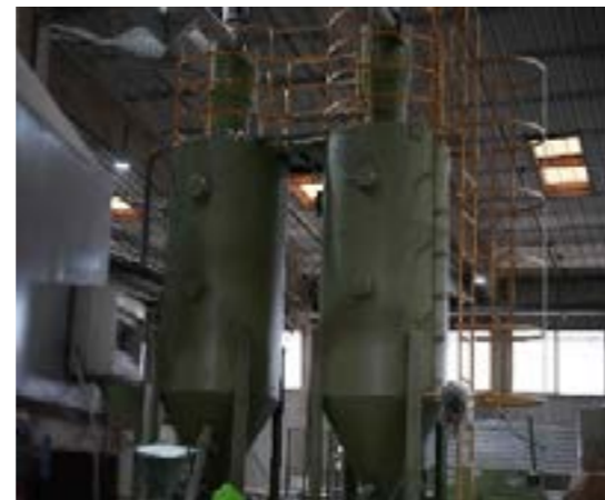
Figure 8. Water Coolers in the Factory
